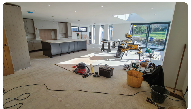
Bespoke kitchen installed in 80M 2 extension
