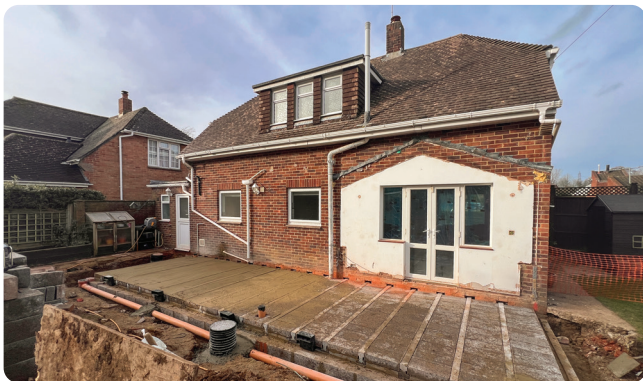
Footings prepared for 30M 2 2 storey refurb
