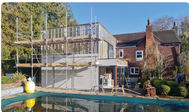
Insulation on 70M 2 extension before cladding
