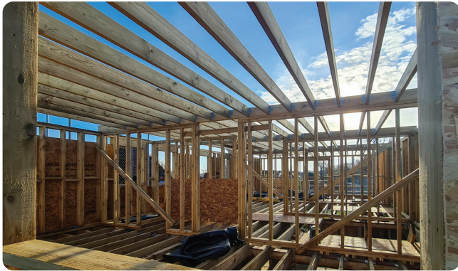
100M 2 2 storey rebuild ready for roofing
