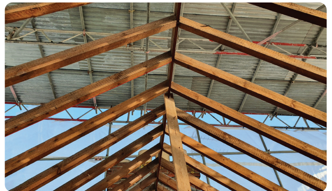
Temporary tin roof protecting loft conversion
